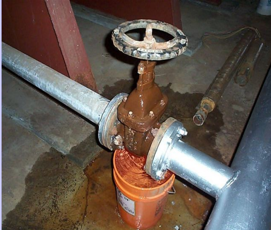
Leaking valve
