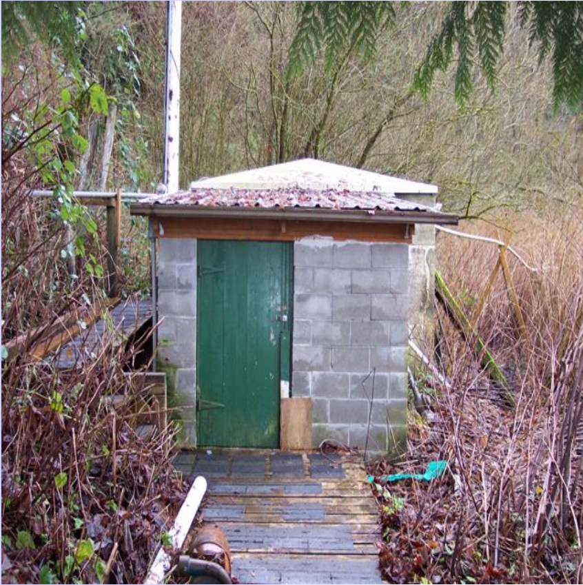
Booster station with above ground piping
