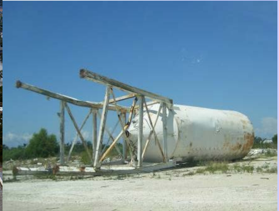
Fallen water tower in Biloxi, Mississippi caused by Hurricane Katrina, August 2005
