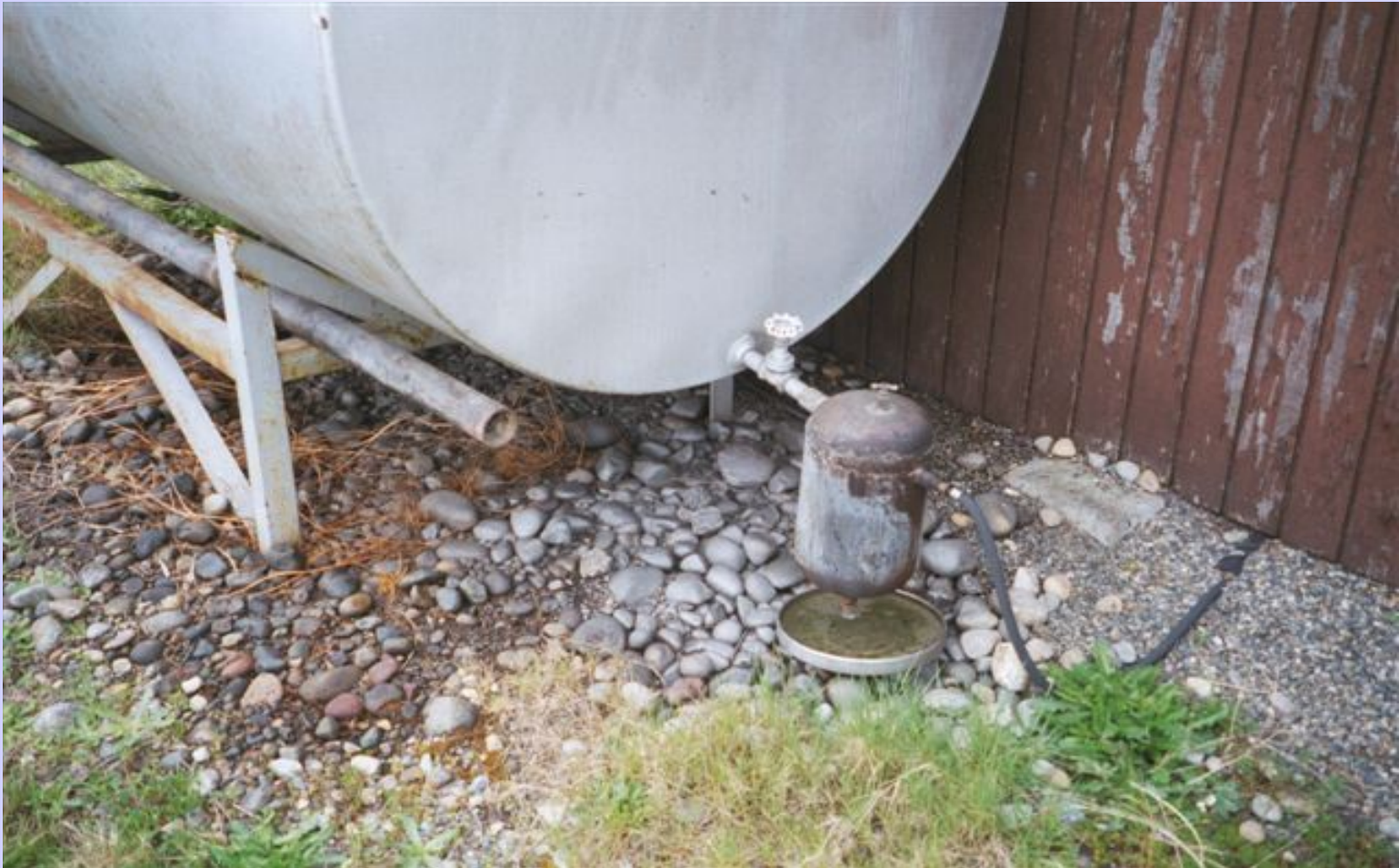
Fuel tank leaking diesel next to wellhead
