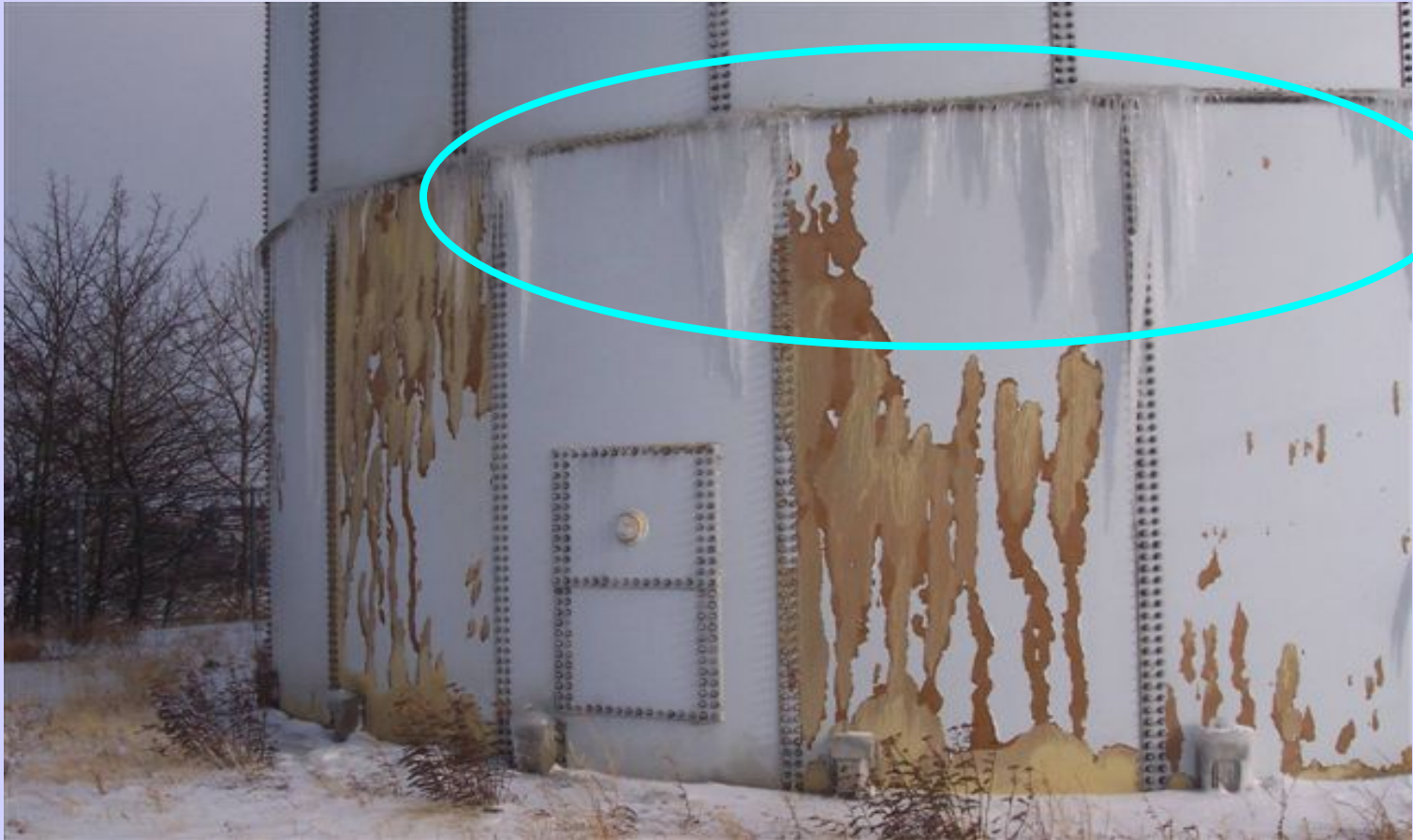
Leaking reservoir
