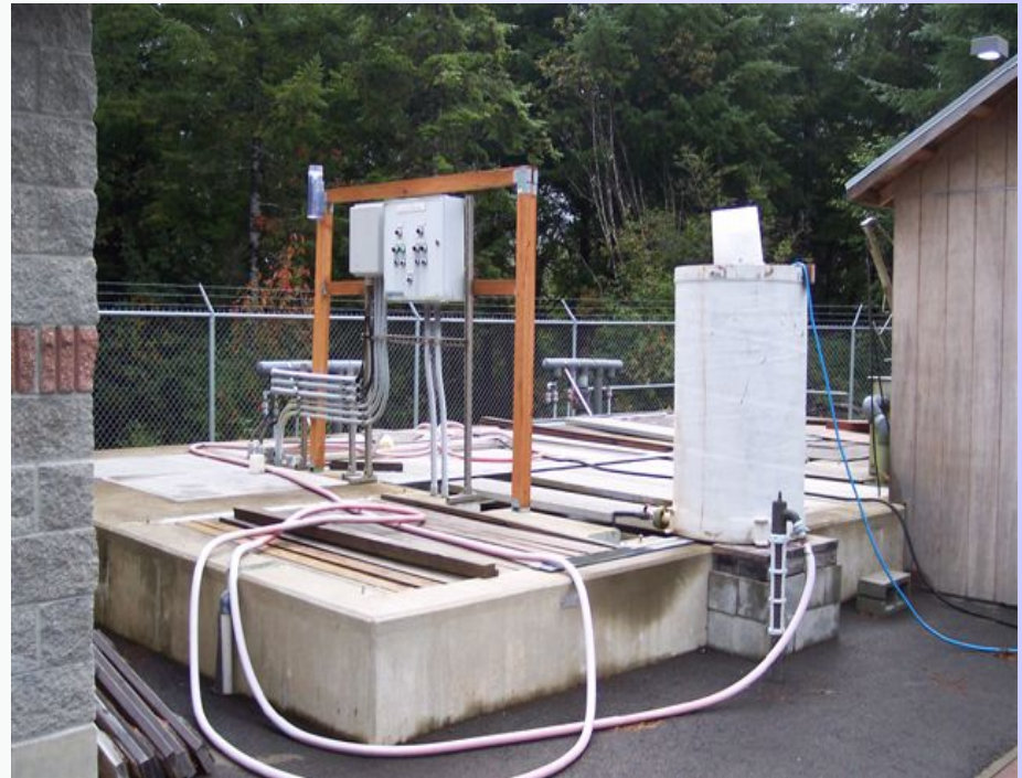
Small wastewater treatment plant
