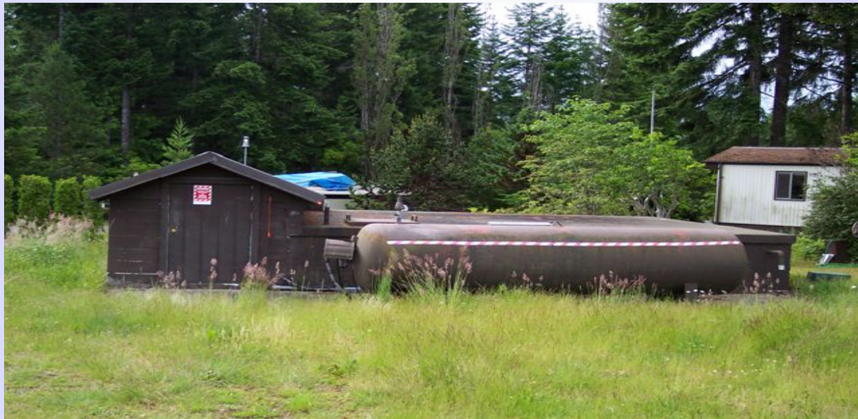
Small system wellhead with hydrotank
