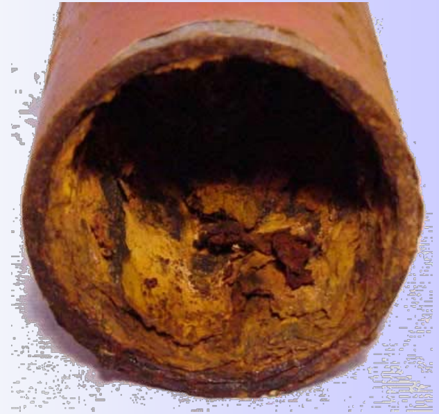
Rusted iron water pipe
