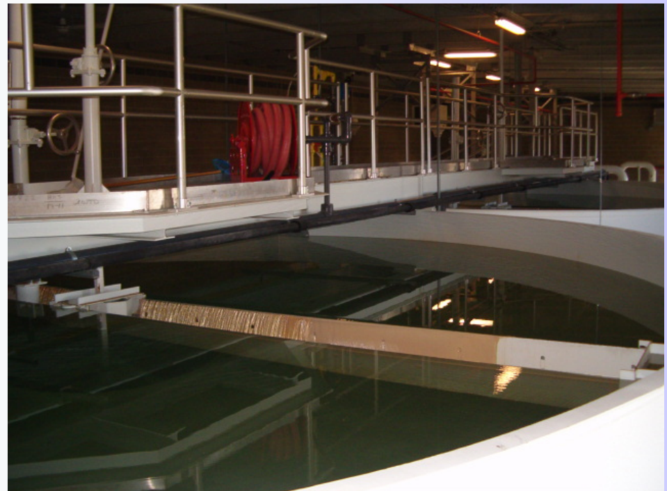
Small drinking water treatment plant
