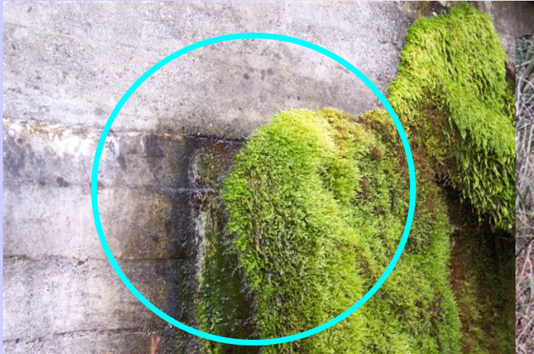
Leaking reservoir wall
