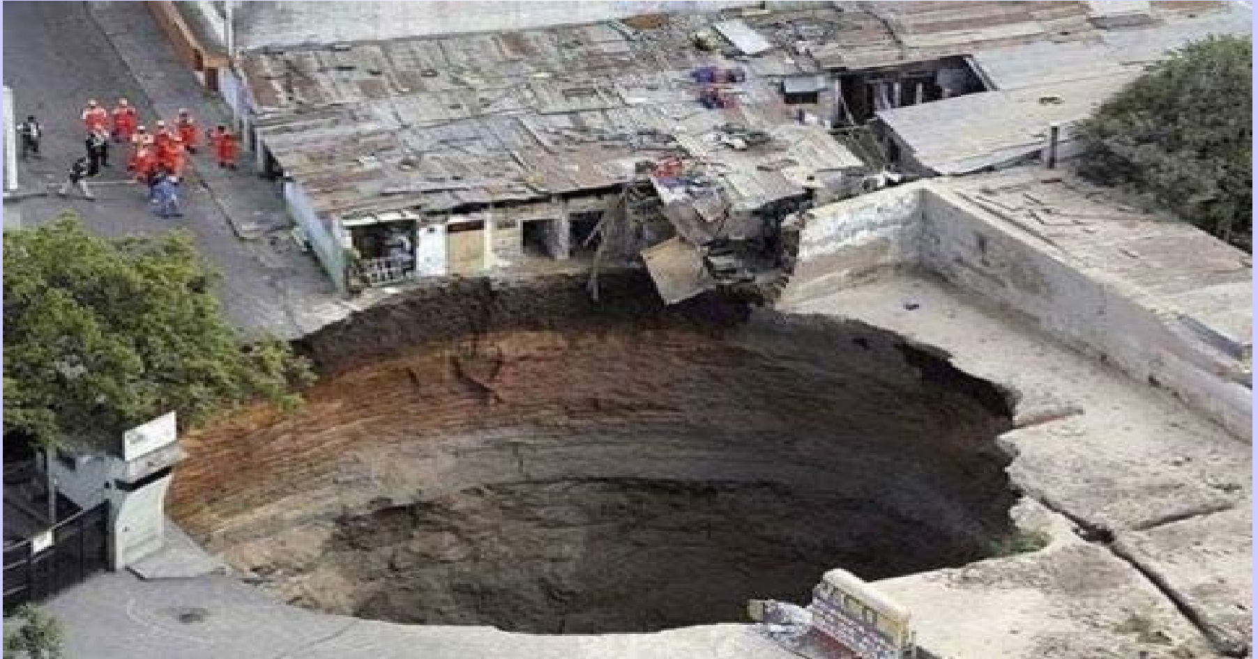
Guatemala Sewer Pipe Explosion, February 2007
