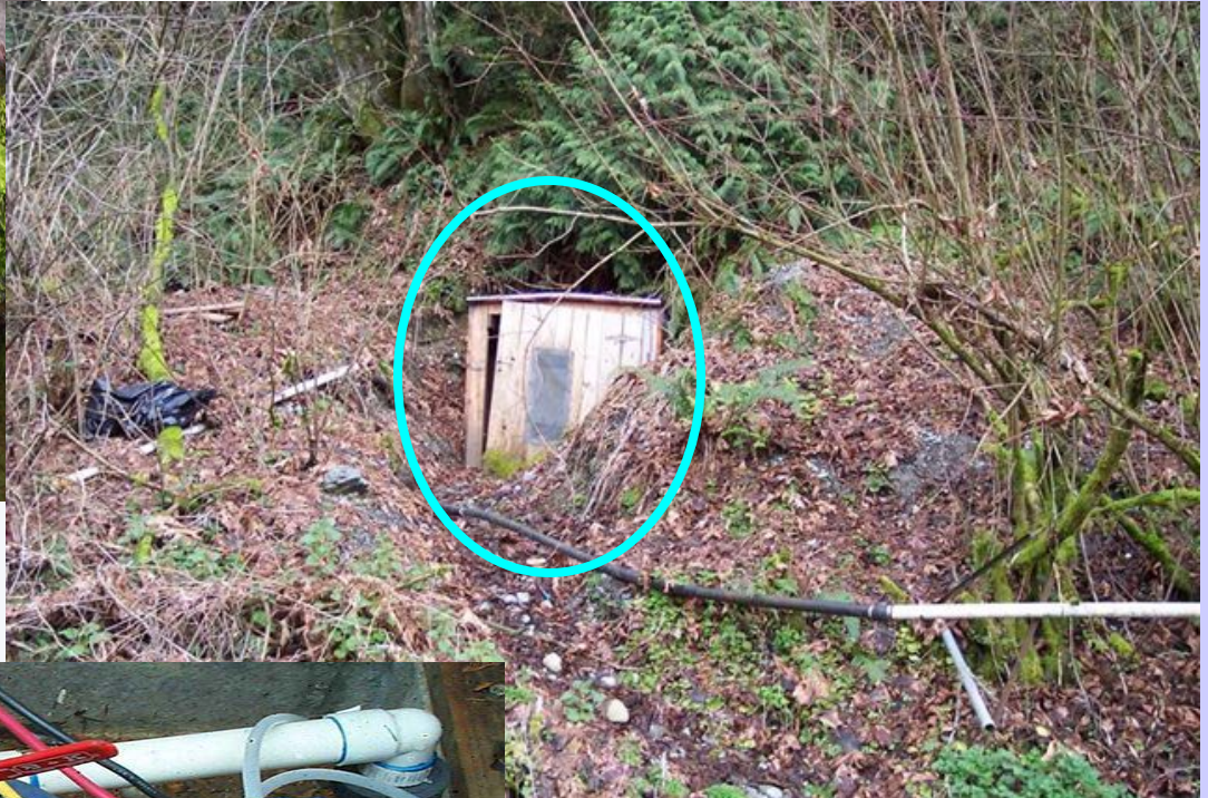
Spring Box with open access
