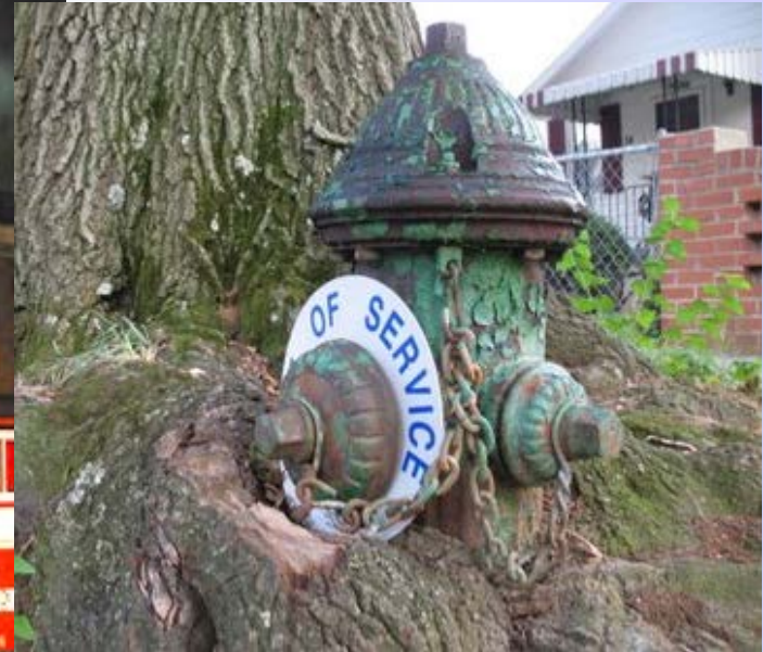
An out of service fire hydrant in DC Credit: Dave Statter, WUSA9 News
