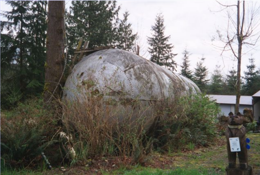
Poorly maintained reservoir
