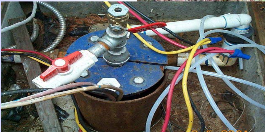
Wellhead that needs to be replaced
